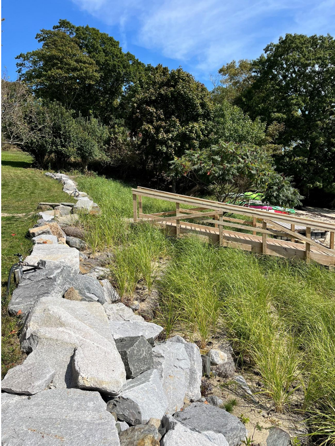
Close-up of artificial sand dune/nature-based solution showing vegetation growing inside coir logs and rip rap on the top.
